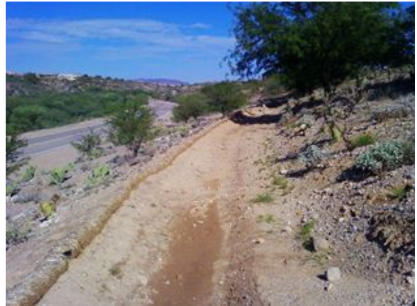
Photo 8. Area 2 – Mid-slope bench/swale with straw waddles looking west.
