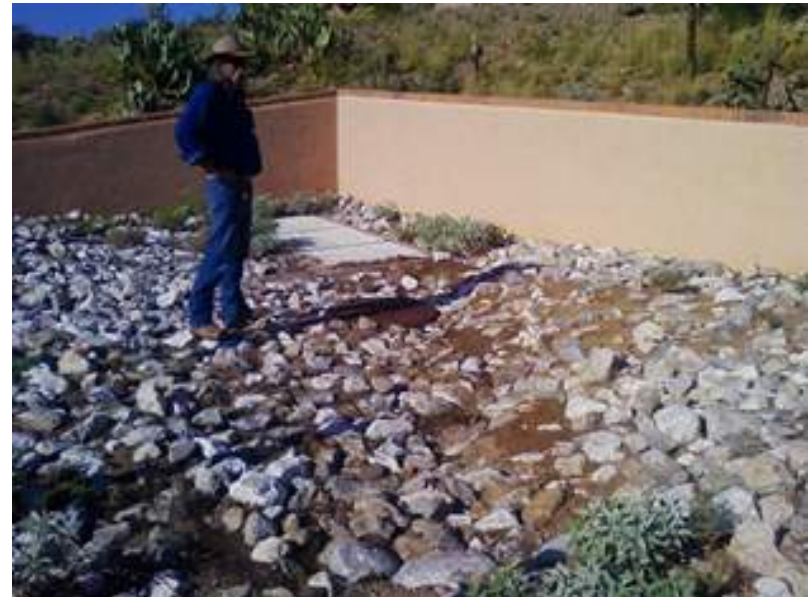
Photo 14. Area 4 – Riprap collection area and area drain – View Ridge Drive at Hidden Crest Court looking west.
